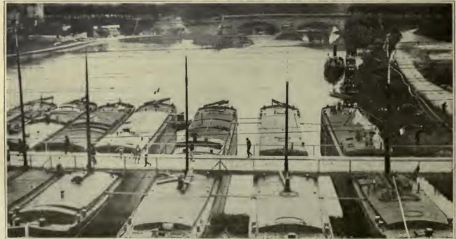
The destruction of bridges by the contending armiss creates a need for other bridges, and as speed in their construction is the essential consideration, they are made of boats or rafts upon which a passage—way is thrown, as shown in this picture.
