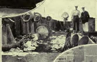
The top picture shows the Carmania; the middle one the wreck of her bridge from one of the Cap Trafalgar's shells; and the bottom picture a hole made in the engineroom casing by a shell that first ripped through a lifeboat and missed the wirelese room on the left by only a few feet.
