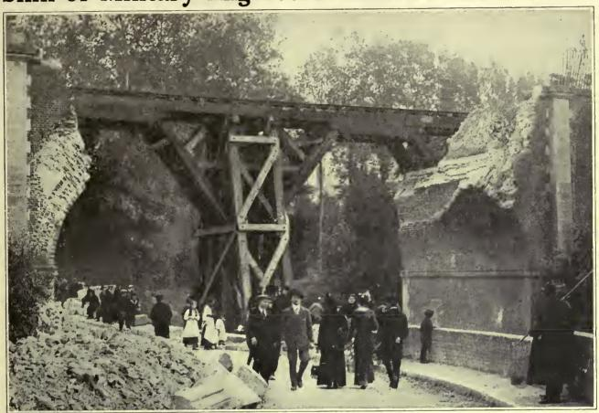
A massive railway bridge of stone and brickwork between Amiens and Rouen was destroyed by Germane during their retreat through France, but British engineers made a strong and serviceable repair with balks of timber, as seen in the picture, thereby restablishing the lines of communication and giving them the use of the railway for the transport of their men, guns, and stores.
