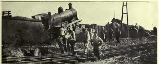
The havor made by the locomotive charge mentioned above was so great that the Germans found it more expeditious to build a new track parallel with the old one instead of attempting to remove the wrecke and repair the old line. This picture shows the new line under construction, with the wheeled chargers in a heap of ruine on the far eide.
