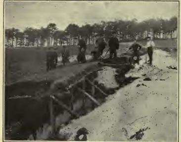
Membera of the Canadian Expeditionary Force working on an invisible trench, the roofing of which coneisted of turf layers aupported by logs.
