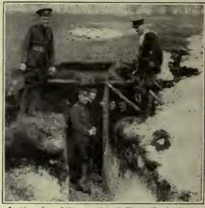
Another view of the same trench, illustrating its depth, and showing how the grass-plot roof hid it from view.
