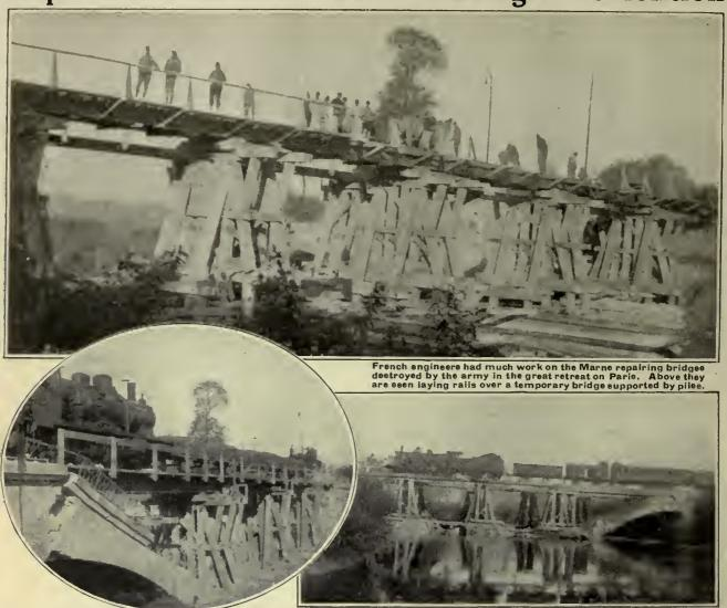
In order to teet the etrength of a new structure a locomotive and trucke laden with ballast are driven over it.
