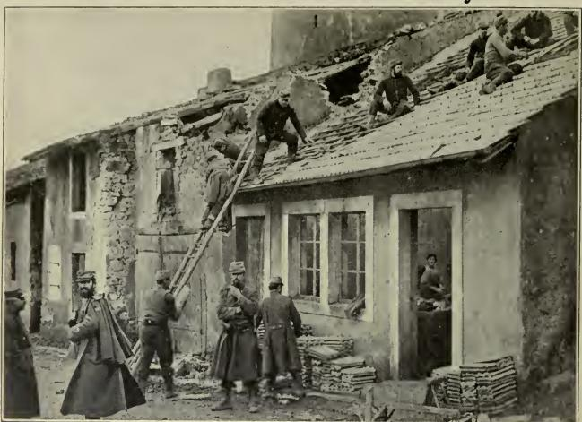
Immediately a village was retaken by the French from the Germane, our allies vigorously set about repairing the damage done by the "Bosches." In this photograph some military engineers are seen at work on the root of a shell-shattered cottage in St. Genevieve, which had not been abandoned by the brave inhabitants, who may be seen at work within the house.
