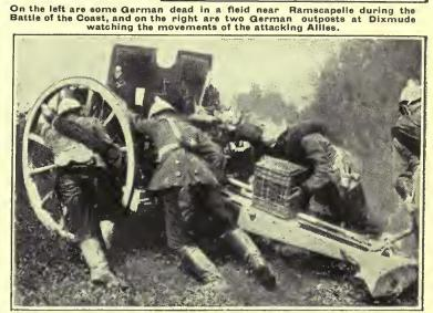
A German field gun being pushed into position. The protecting shield and the hole through which the gun-layer sees the objective will be noticed.
