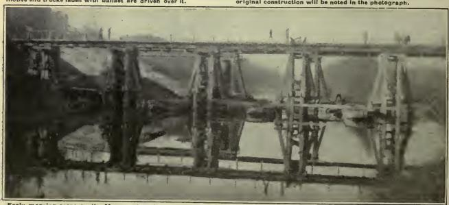
Early morning ecene on the Marne, when the only dieturbance was the hammering of French engineers. The above photographe are exceptionally interesting as showing the ingenious and rapid work of the French engineers, and were taken by a soldier in the 7th Company of Engineers. Most of the bridges blown up in this district were speedily replaced with temporary structures.
