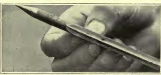
Ths "fischette" is a small steel arrow used by Frsnch, Russian, and German aviators. When dropped from above on an unsuspecting soldier it could pierce hie body from head to foot.
