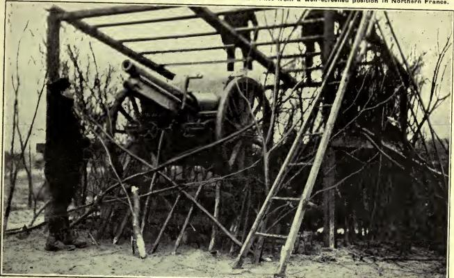
Hiding the terrible "75." Belgian artillerymen erect a wooden shed round their gun, completely masking it from all points of view. Only the extreme etability of the "75" in action makes each complete cover possible.
