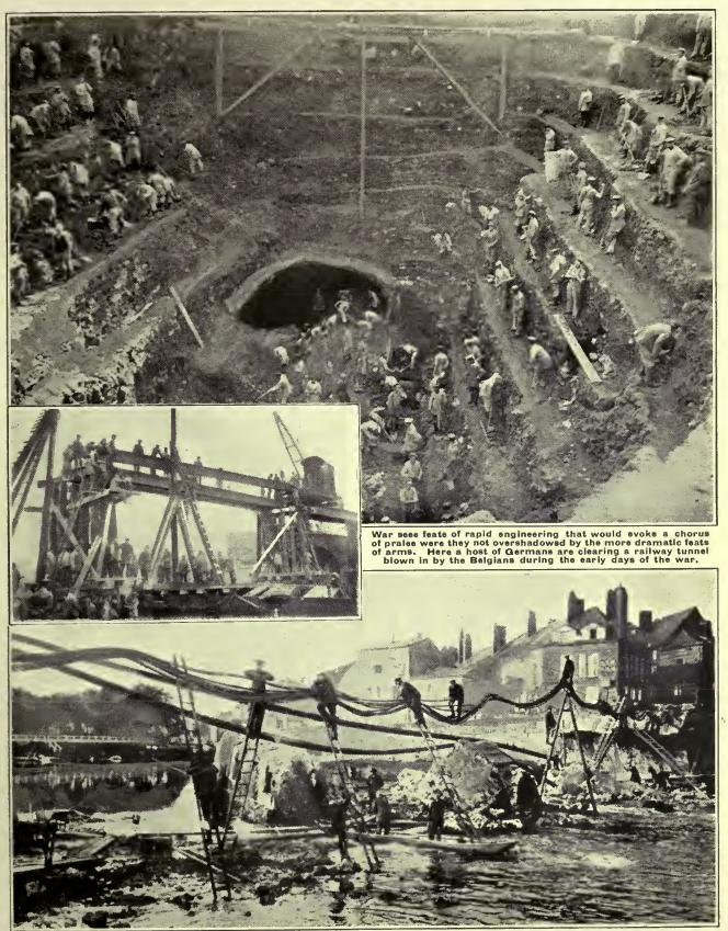
German engineere beginning to repair telegraph and telephone cables left, as shown, when the Charleville Bridge was blown up.
