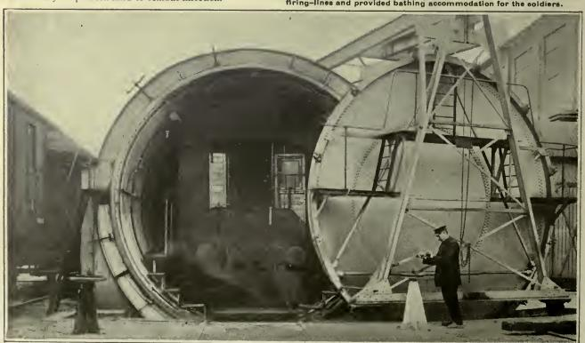
Another view of the remarkable apparatus installed at Potedam, in which an entire railway coach can be thoroughly disinfected. The coach inside has been used to carry infectious "cases" from the front, and, in order to safeguard against infection among the troops, is about to be disinfected before being put into commission again.
