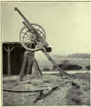
So slight le the recoil of the "75" that it is possible to balance it on an improvised wooden tripod in order to use the weapon as a high-angle anti-aircraft gun.
