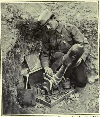
Firing a torpedo of the air from a 58 mm. trench-gun. The projectile was "winged," weighed about thirty-three pounds, and could be fired a distance of nearly aix hundred yarda.
