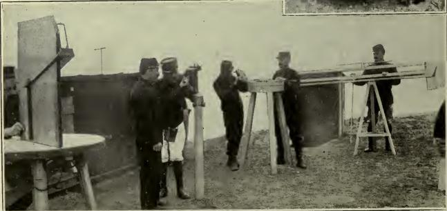
Many inventions of uss in connection with foiling hostils aircraft rendered service in and around the city of Parls. This photograph shows one of the anti-aeroplane observation posts, fitted with instruments for gauging the height, dietance, and epeed of
