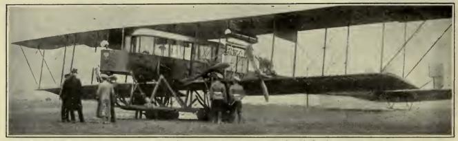
Largest biplane yet invented. The gigantic Sikorsky machine, a feature of the Ruseian Air Service, which is driven by four 120 h.-p. engines working four separate propellers. The biplane is fitted with a large cabin designed to carry as many as twenty persons.
