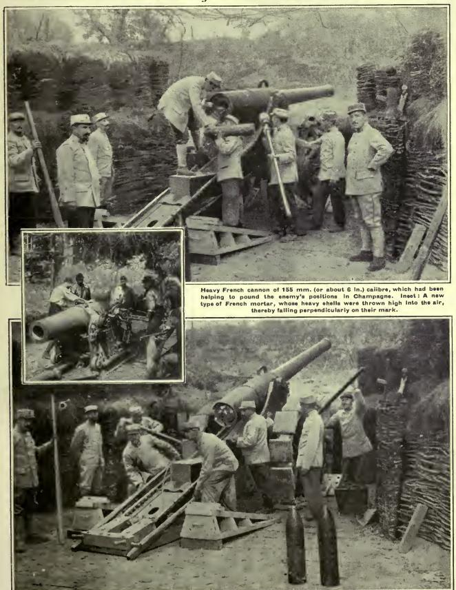
Immediately after the recoil. The sequel to the first picture on this page, showing the 155 mm. gun being hauled into position again for another shell. Note how the emplacement is surrounded by watties covered with grass, which give the appearance of a high hedge.
