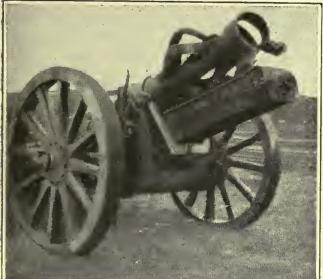
Literally torn to ribbons. The barrel of a faulty German gun which exploded, killing the gunnere instantaneously.
