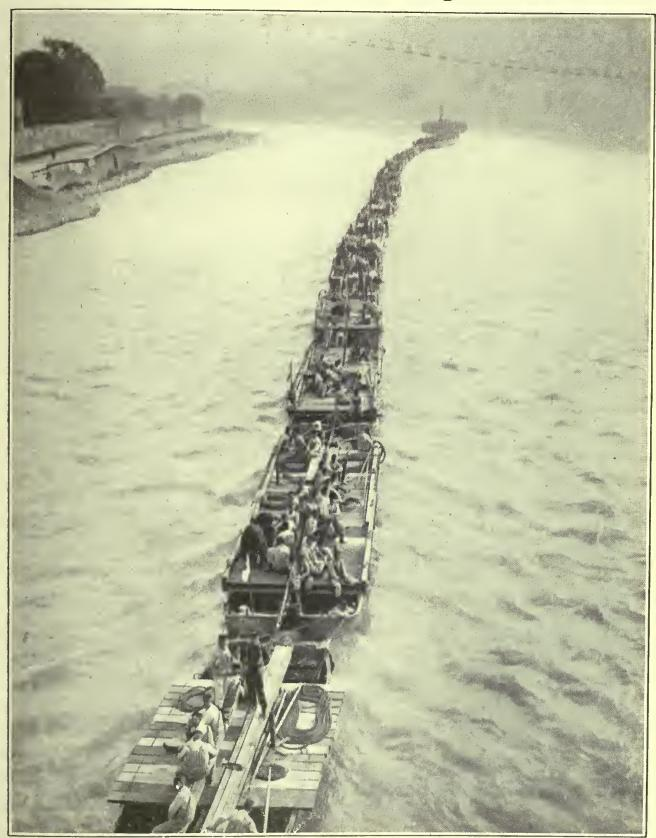
French military engineers on a long pontoon bridge that ie being towed up a river to its poeition. The bridge is practically completed, but it ie in esctione, which are connected when they have been swung into the required poeition acrose the etream.
