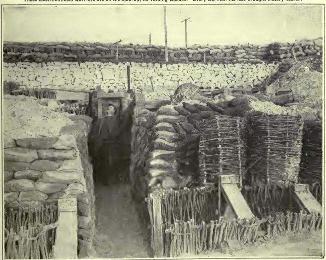
How a French artillery commander's hsadquarters wers made more or less immune from destruction by enemy shelle. with which the poeltion was consolidated with stones, sandbage, loge of wood and gabions is characteristic of French thoroughness. Nothing less than a powerful mine could shatter this very strong dug-out.
