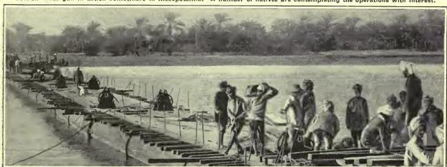
Indo-British pioneers constructing a floating bridgs across the Tigris. The rapidity with which these quite substantial constructions are completed le one of the marvels of modern campaigning. During the war doubtless more bridges were destroyed and built than at any other period of time in the world's history.
