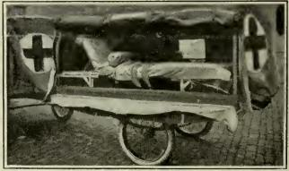
Motor-drawn German Red Croes waggone of a new type. As illustrated in the right-hand photograph, the canvas sides and ends could be rolled up, allowing ambulance workers to attend to the wounded without having to remove the men, and also obviating the dreadful joit that could not be avoided when the stretchers themselves were pushed head-first into ambulances.
