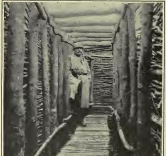
Neatly constructed French trench. A wood flooring was laid down and the walle were consolidated with watties.
