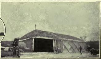
Portable naval hydropiane hangar. These invaluable shede were erected and taken down with remarkable rapidity.
