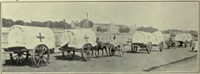
Red Cross ambulances for use in the Desert of Sinal. They are fitted with broad wheels to prevent their sinking too deep into the sand, and have a spring flooring constructed on the principle of the wire-mattress.
