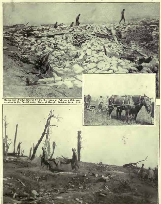
Bringing in wounded across open ground at the edge of the forest. Inset: French soldiers laying an underground telephone cable. The apparatue ploughs a furrow along which the reel laye a cable. The furrow is then filled in by an inverted sloughehare behind the reel.
