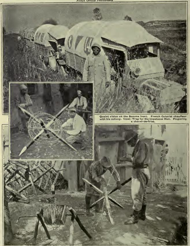
Beginning of a cheval-de-friee to consolidate a newly-captured position. Barbed-wire le coiled round three etakes, and a number these obstructions are placed together to form what le the most formidable defence work available in a short space of time.
