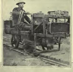
"SCOTCH EXPRESS" IN FLANDERS .-- Light railway engine constructed from parts of a tnset: Conveying raile to lengthen the transport line just behind the British front. (Official photographs.)
