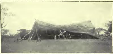
Portable aeropiane hangar at Serengeti Camp, showing a machine at reet.
