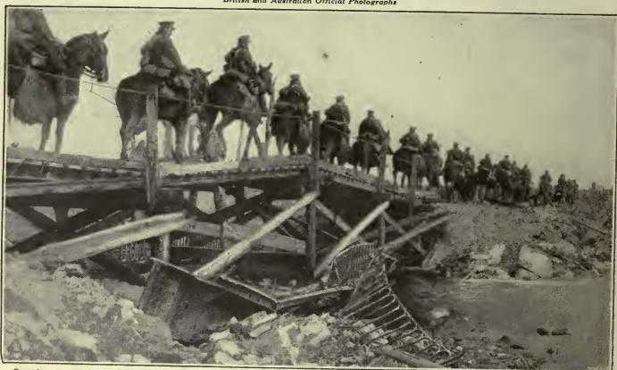
Crossing a rapidly-made bridge in the wake of the retreating Germane. Though the enemy was careful, by destroying bridges and damaging highwaye, to impede their pureuers, the advancing British lost no time in making the bridges usable again.
