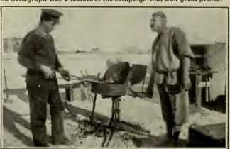
A native working the bellows of a portable forge being used in the desert by a blacksmith of the Royal Engineers.
