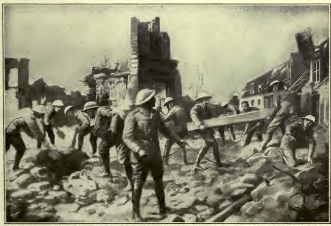
Making good the roadway in a wrecked village whence the enemy had been driven. The pioneers worked steadily with pick and shovel, despite shell fire, while the officers taped out the road "as though taking up the Strand in the good old days before the war."
