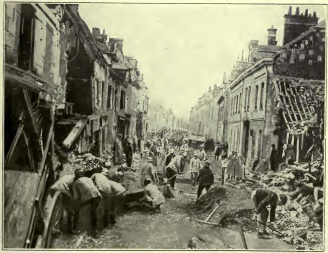
French engineers repairing the Rue de Parie in reoccupied Noyon. The retreating Germane mined large holes in the etreets to hinder their pursuers, but when the French reached the town they promptly eaw to the levelling up of the craters.
