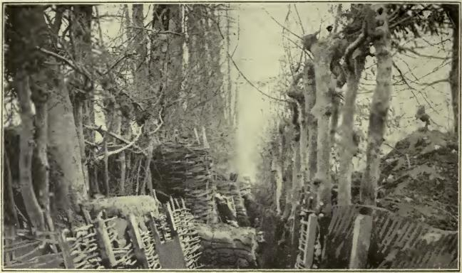
Well-planned and carefully-contrived British trench used during the 1917 advance on the western front. It was so arranged as to seem a bit of woodland, the tree-trunks forming not only supports for the parapets but serving to shelter the men from observation.
