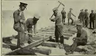
Men of the Egyptlan Labour Corps—Arabs and fellaheen—making a cutting for a railway, and (right) a railway company of the Royal Engineers driving in spikes of a new line. Decauville rallways and lines of metre gauge supplemented the standard-gauge lines.
