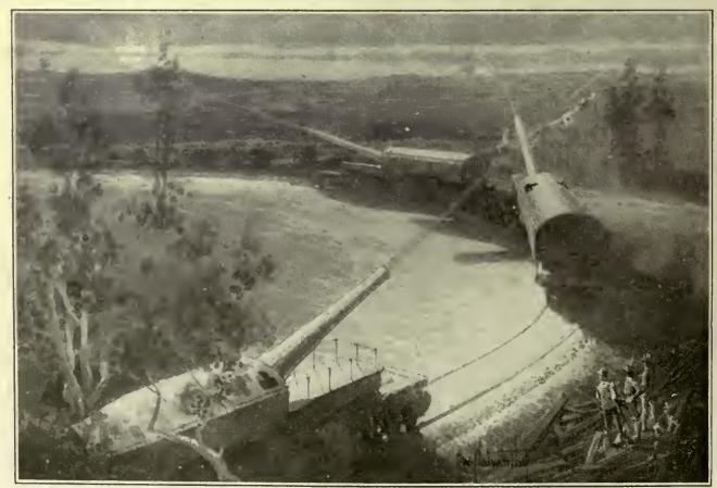
MAVAL GUNS IN ACTION ASHORE.—Long-range naval guns were used with affect on the Somma. Owing to their length of barrel they can only be fired on the axis of the truck, and to lay the gun the truck is moved backwards and forwards along raile laid in a curve
